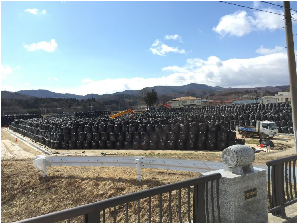
988 Figure 6. Temporary storage facilities for radioactive waste in Iitate Village, in the Fukushima 989 Prefecture.
