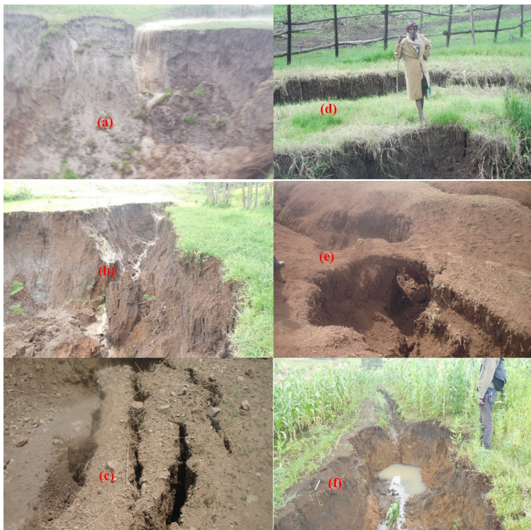
Fig. 7. Examples of gully expansion controlled by: (a, b) bank geometry (height and slope), (c) tension cracks, (d) land slide, (e) soil pipes and (f) saturated vertisols (gully development on conservation ditches, narrow ditch upstream of gully headcut) in the sub-humid Debre Mawi (a,b,d, and f), Mota (c) and Geregera (e) watersheds (pictures taken in 2013).
