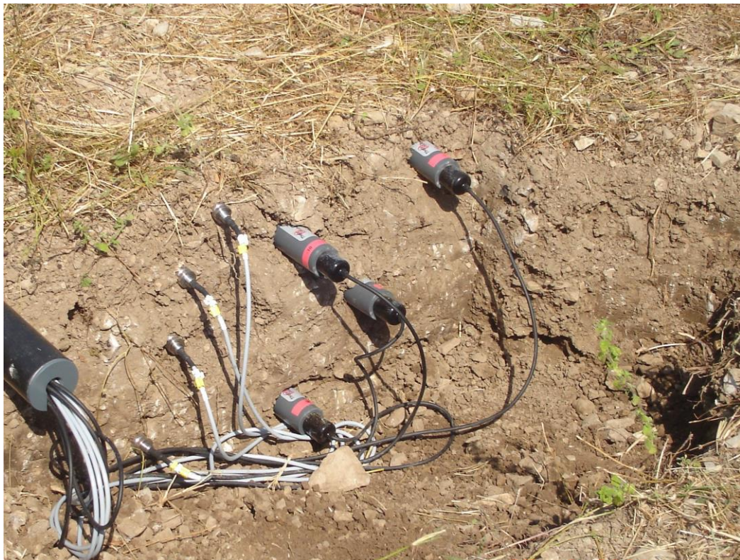
Figure S1.9 - Installation of the probes at Prades-le-Lez (PRD).
