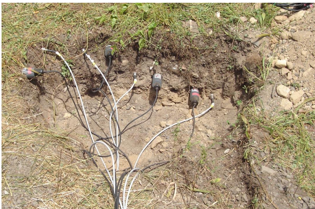
Figure S1.7 - Installation of the probes at Barnas (BRN).
