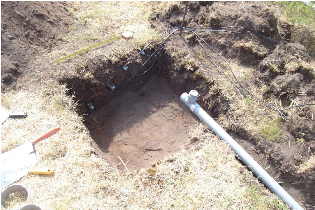
Figure S1.5 - Installation of the probes at Sabres (SBR).
