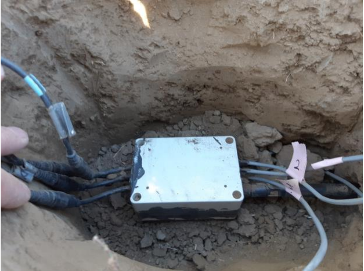
Fig. S8. Field installation of the underground node.
