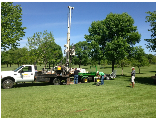
Figure 2. Soil sampling and monitoring well installation at East 18 course.
