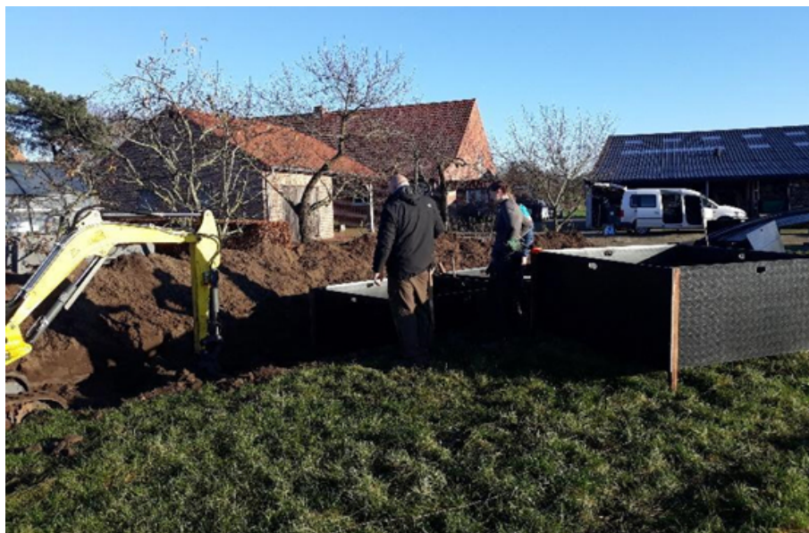
Figure A6. Excavation works during set up of experimental site, showing the black impermeable plastic boxes and the crane used for de-compaction.
