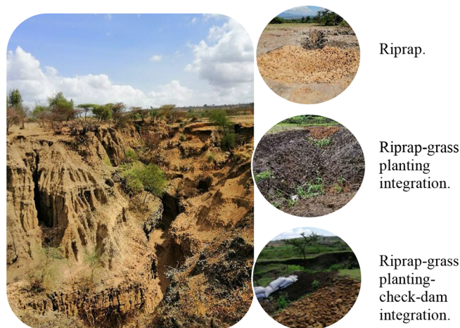
Figure 2. Severe gully erosion in Aba-Bora and low-cost mitigation options. Picture credit @Wolde Mekuria.
